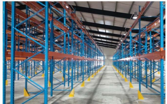
The racking system was installed - with barrier protectors and end protectors to minimise fork lift truck damage in the future - over a period of two-weeks. Dempson were able to move in to their new warehouse in a tight timeframe minimising disruption to business continuity.
